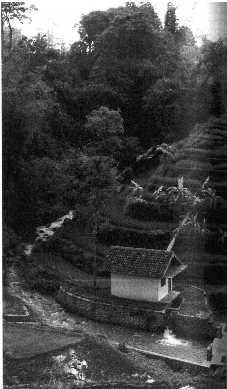
New and old technologies: The terraced rise fields of Seloliman on East Java provide a scenic backdrop for a 12 kW mini hydro power plant.
